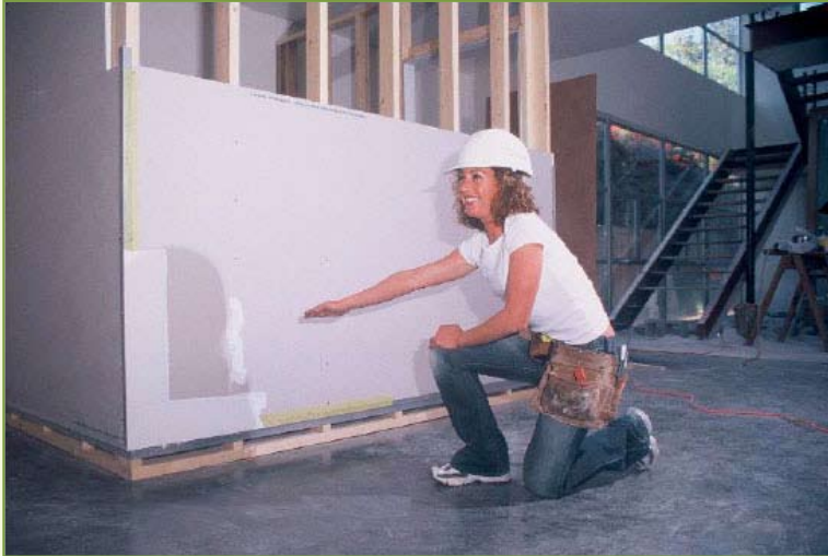
Figure 5-14: Tape and finish the rest of the drywall conventionally.
