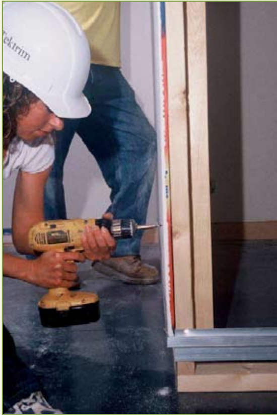
Figure 5-6: Fasten the drywall to the framing conventionally.
